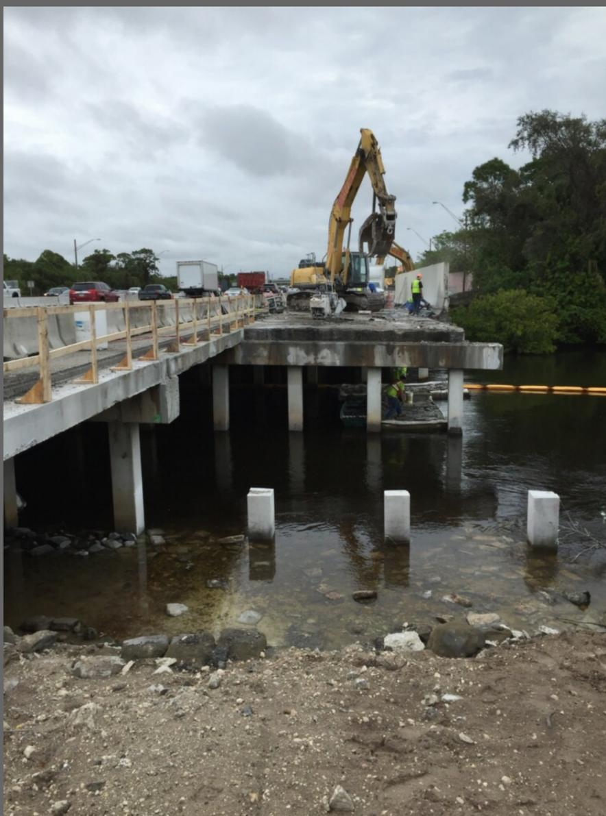
Here we are removing the remaining concrete pile caps & columns on the bridge.
