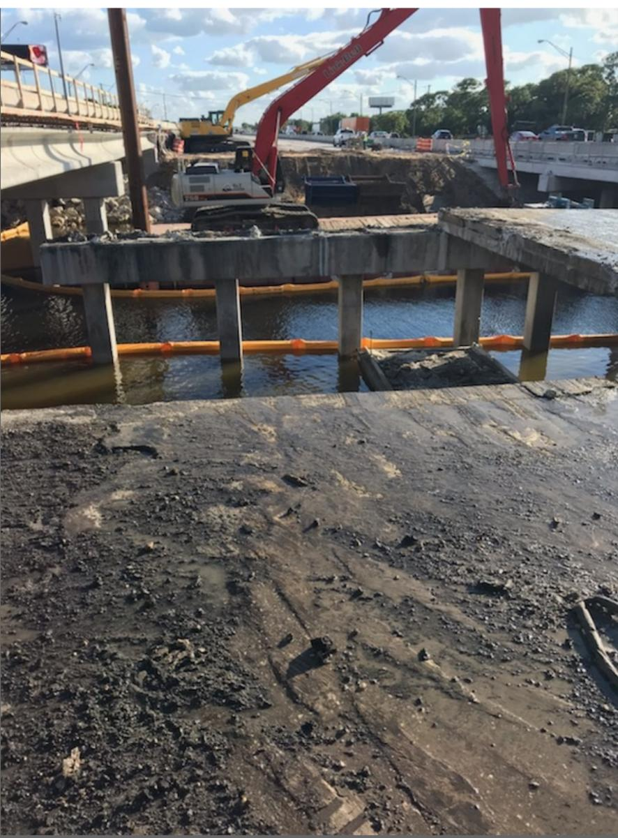
Due to the active waterway below & the multi lane expressway on both sides of the bridge, the removal was performed using specialty wire saw concrete cutting, torch cutting from barges & the use of deep cutting concrete saws.
